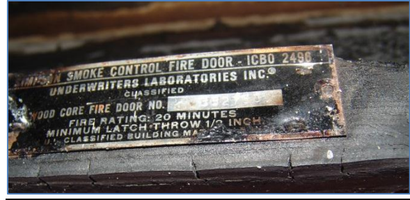
Figure 6: Door plate, fire rating 20 minute particleboard core
