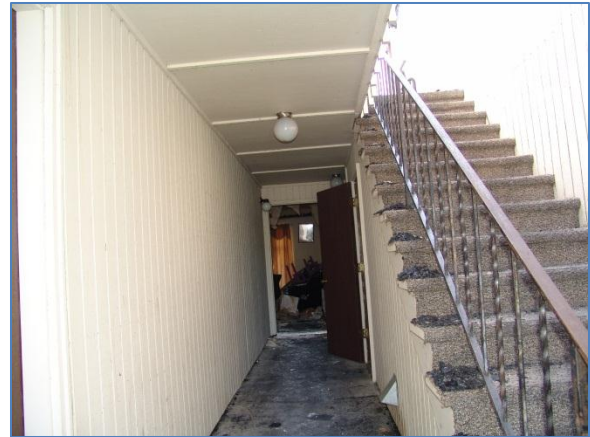
Figure 3: Exemplar structure central corridor and stair. Laundry door under stair.
