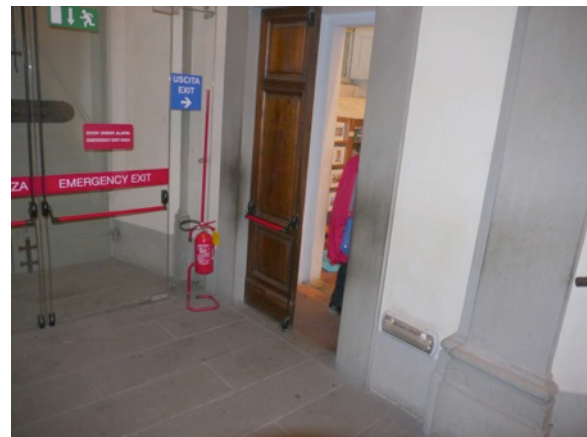
Figure 8. Uffizi Gallery, Florence: if the bookstore is on fire this door is the only barrier to effluent spreading up the primary exit stair from the collections.
