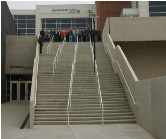
Figure 2. Regulators approved this exit funnel based on a mathematical exit analysis that simply ignored the problem of crowd crush.
