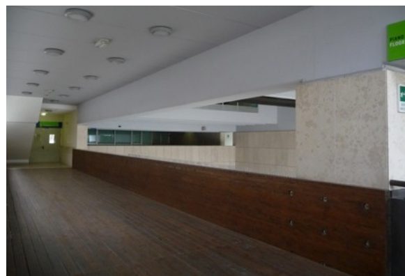
Figure 15. Centro Culturale Candiani, Mestre (recently completed). Very complex building with a cinema, showrooms and offices. External emergency exit walkway made entirely of wood instead.
