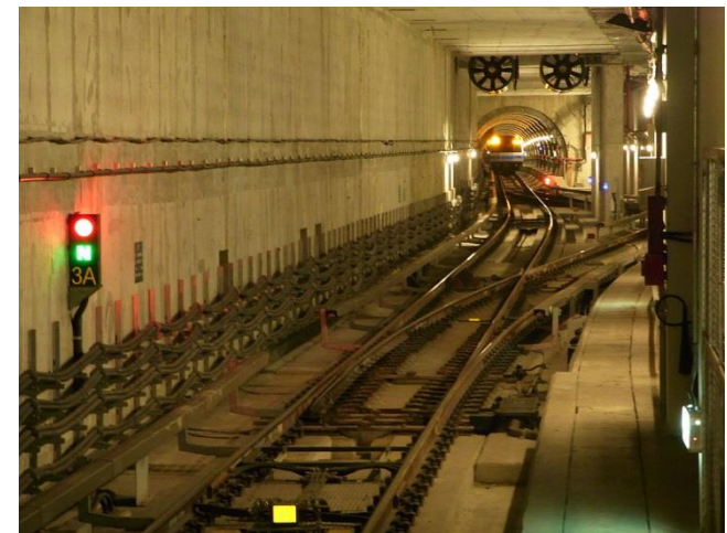
Source: https://en.wikipedia.org/wiki/Tunnel#/media/File:A_crossover_on_the_south_side_of_Zhongxiao_Xinsheng_Station.JPG Accessed 2016/10/19, reproduced under GNU Licence V 1.2.
