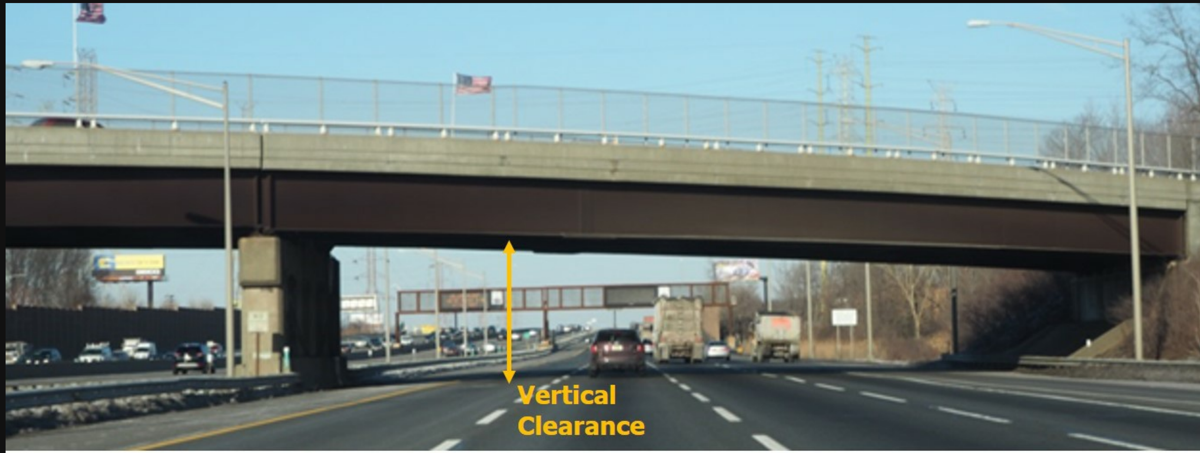
Vertical Clearance (6 and 9 meters)
