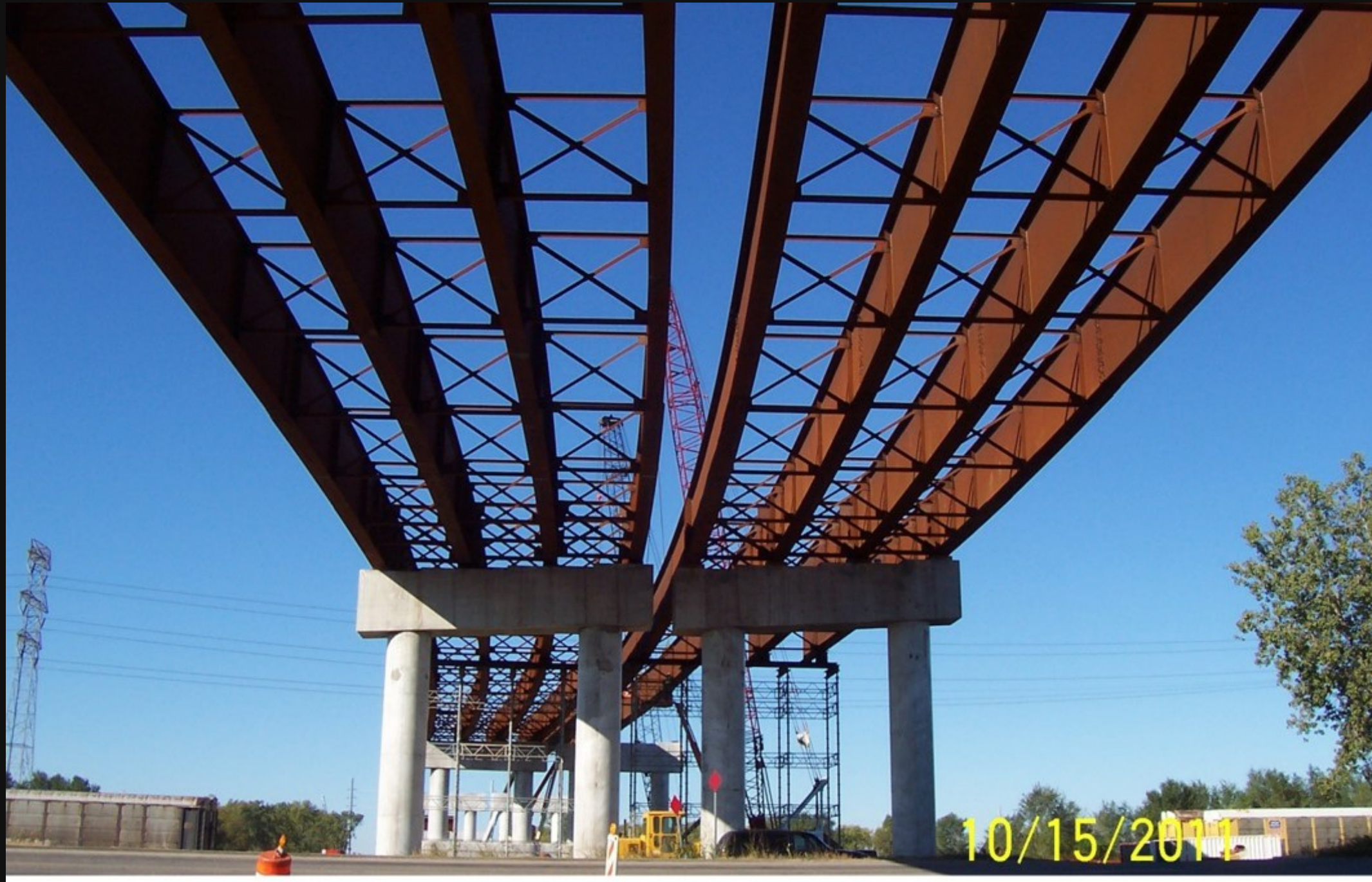
I-Girder bridge construction
