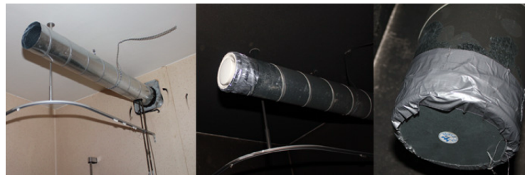
Figure 6. Ventilation system configurations. Open, normal, and closed.
