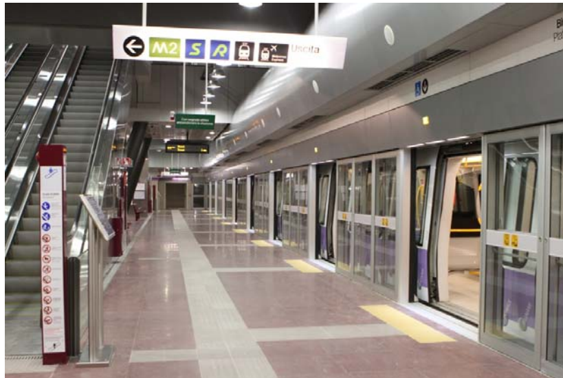
Figure 3.d. – Exhaust grids in the M5 subway line in Milan (Italy).
