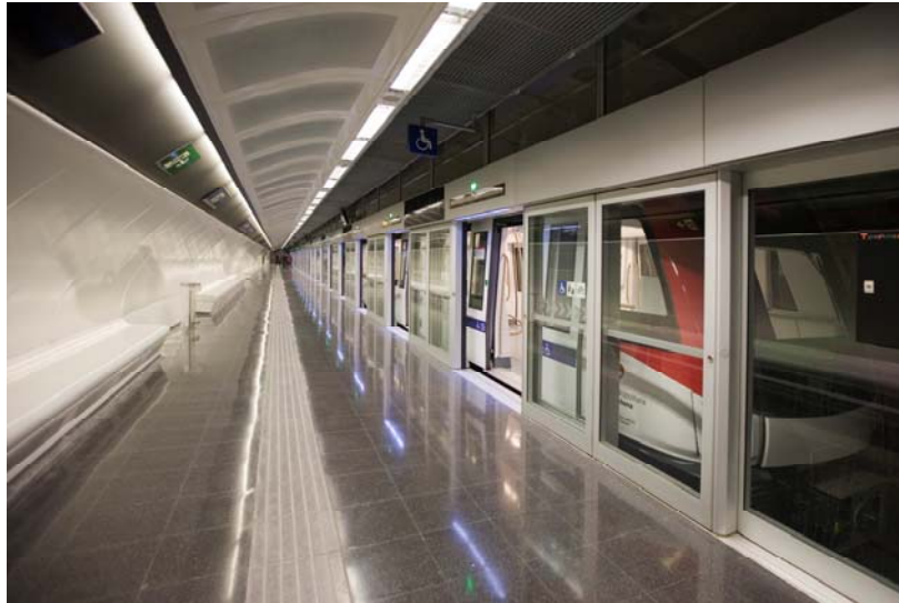
Figure 1.a. - Platform Screen Doors in Barcelona's subway (Line 9).
