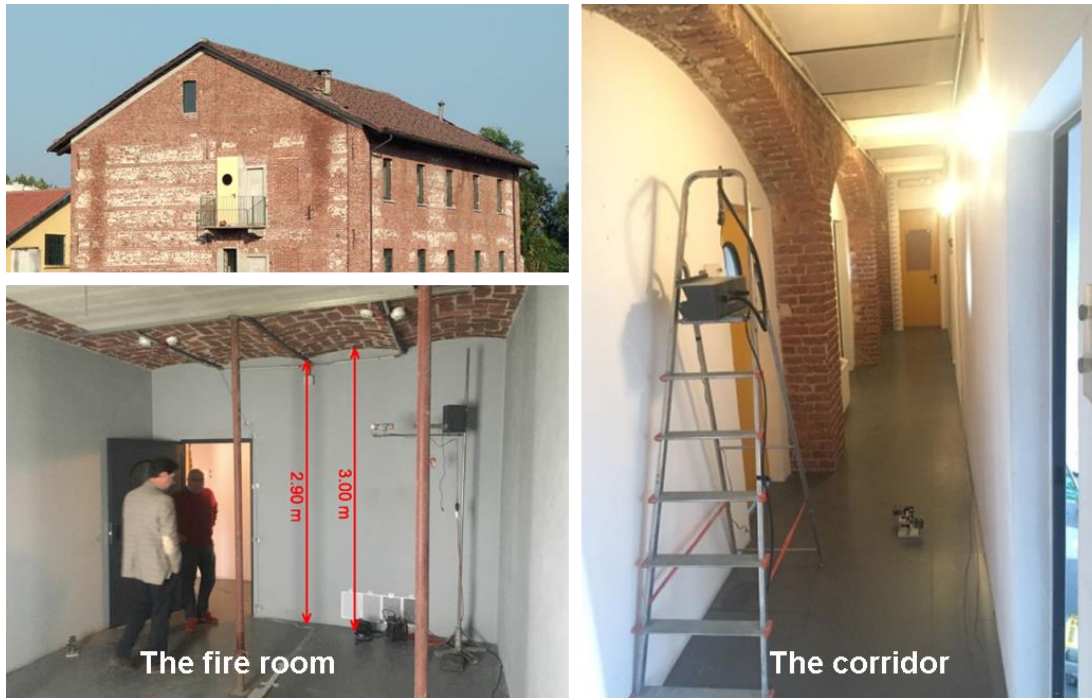
Figure 1: The building used for the experiments - photos
