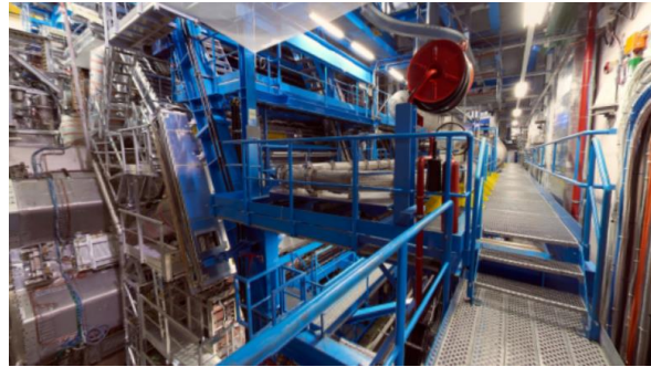
Figure 1 Detail of the escape routes with grid floor on the right and the detector on the left (see stairs and narrow passages)
