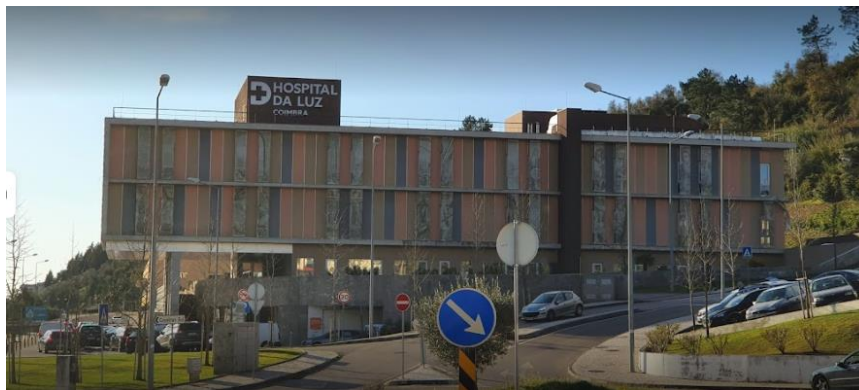
Figure 1: Illustration of a lateral facade of the Hospital da Luz Private Clinic
