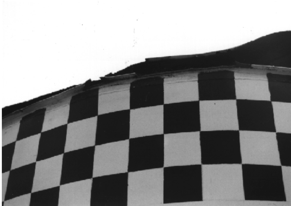
e: Failure Occurred on Roof Plate and Top Angle
